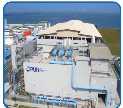
Water Desalination Plant
