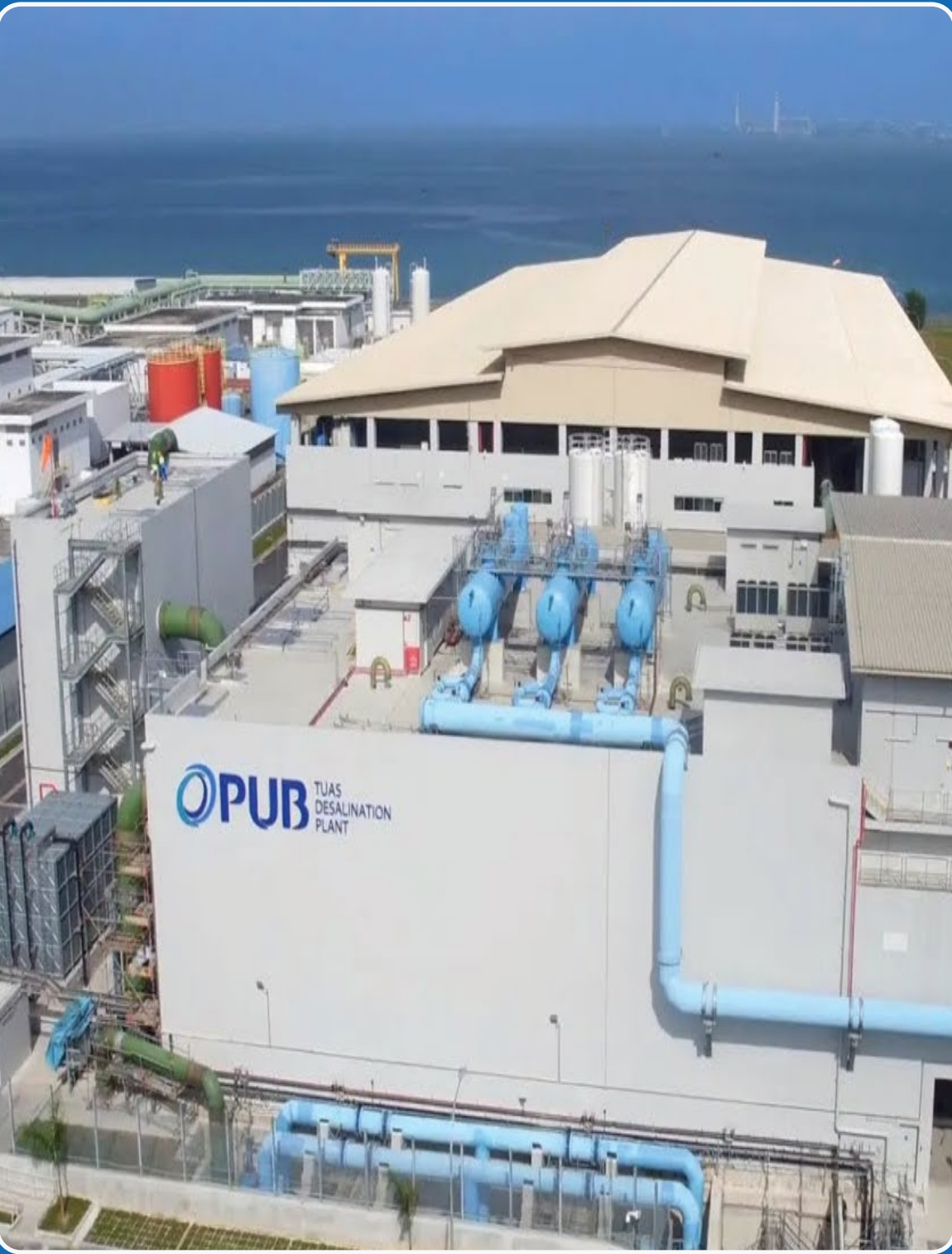
Water Desalination Plant
