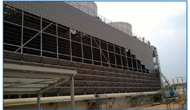
FRP Structural for Cooling Tower
