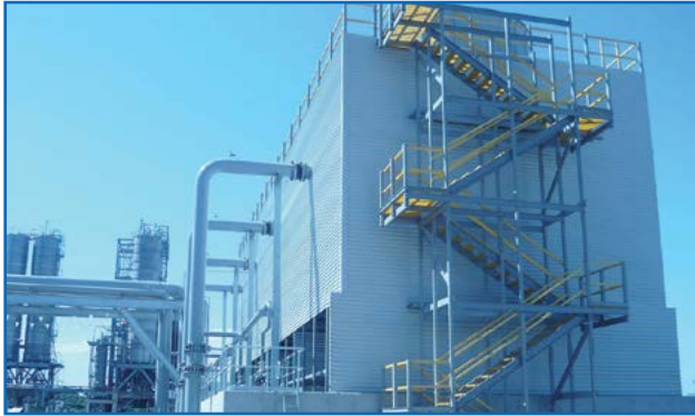
FRP Structural for Cooling Tower
