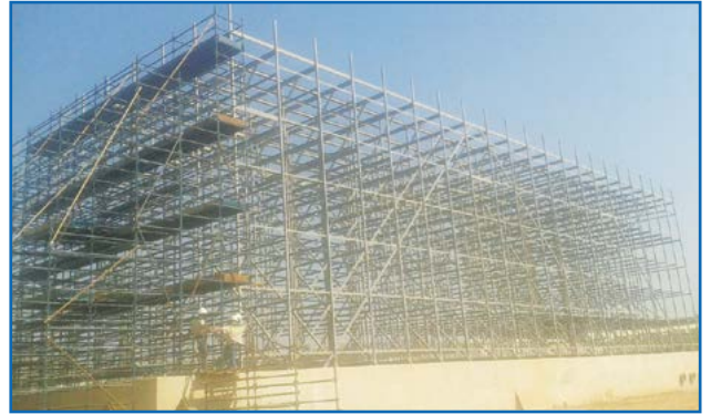
FRP Structural for Cooling Tower
